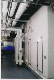
Similar noise-attenuating panels are installed in the ductwork connected to the air-handlers.
