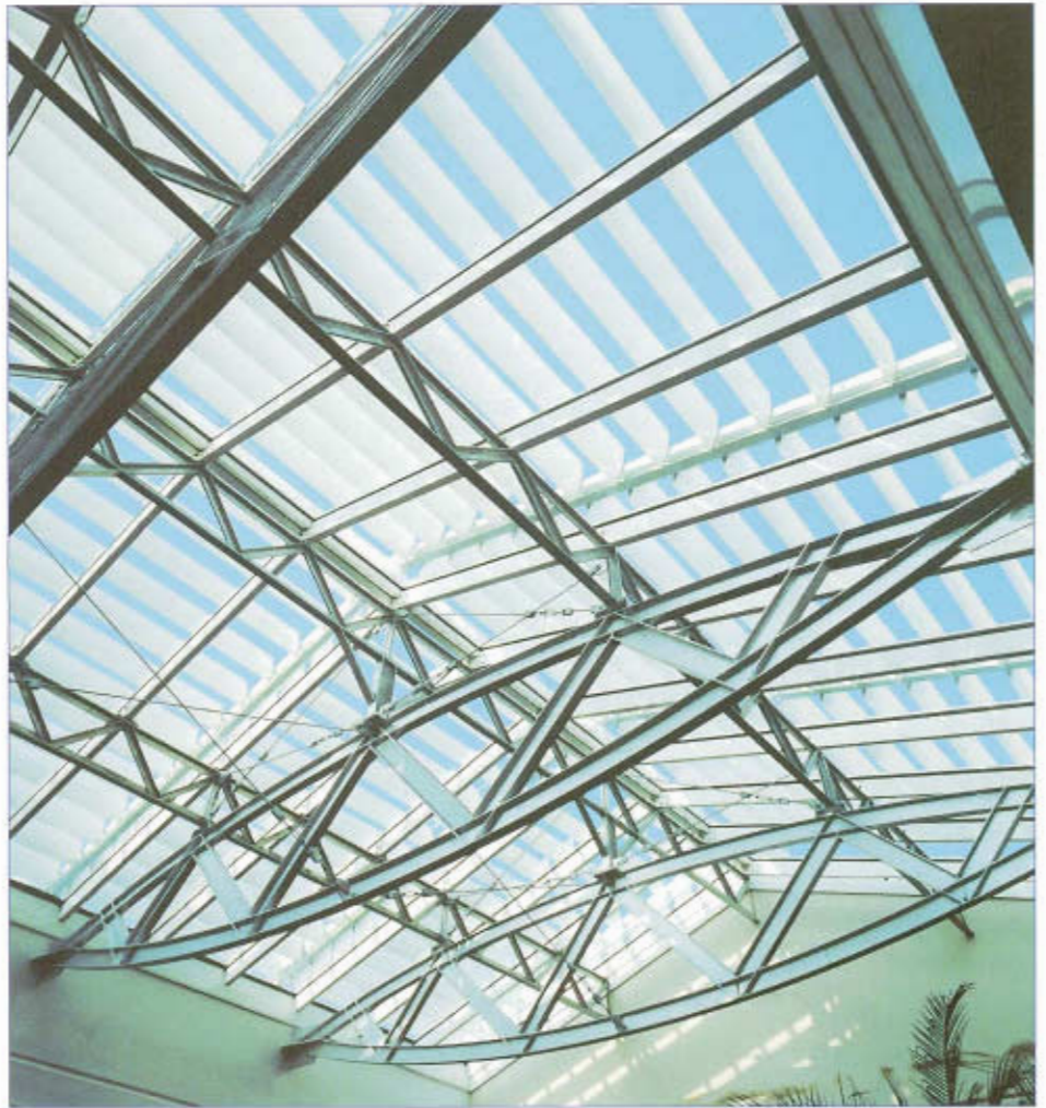
Above: Main offices of SEMAG in Milan with the use of sunbreakers type 30 NT in white, on external support brackets.
