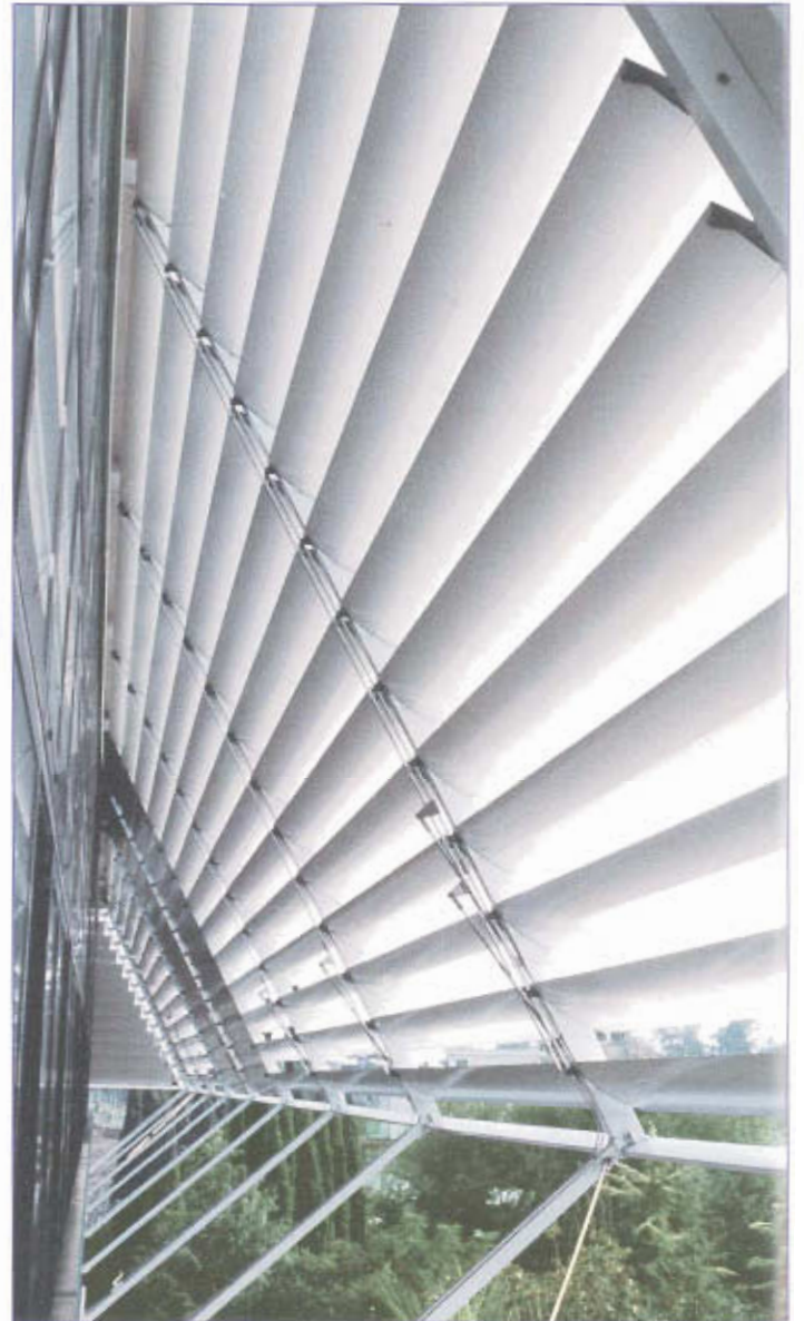
Three photos of an ERG petrol station, with annexed café and halls in Salerno. The type of sunbreaker used is type 30 NT, colour white.
